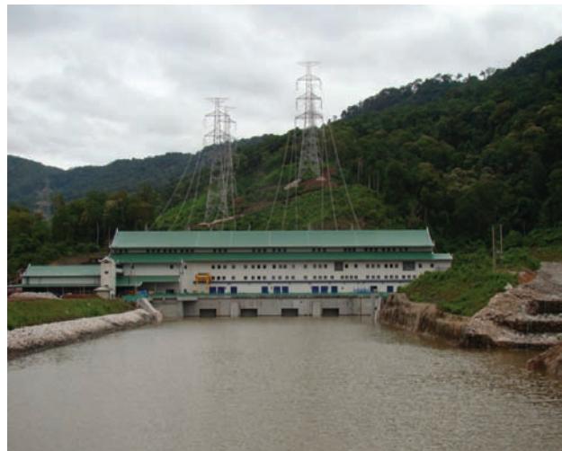
Photo 2: View of Powerhouse
