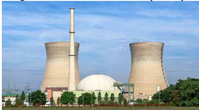
Fig 1: A nuclear power station (Grafenrheinfeld Nuclear Power Plant, Grafenrheinfeld, Bavaria, Germany). The nuclear reactor is contained inside the spherical containment building in the center - left and right are cooling towers, which are common cooling devices.
