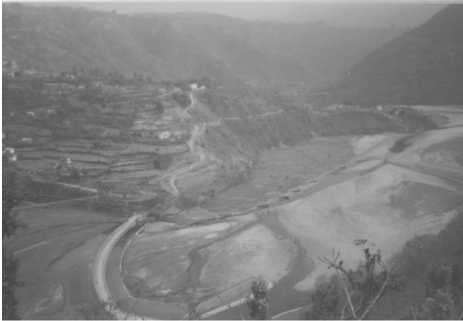
12MW Jhimruk Hydropower Project
