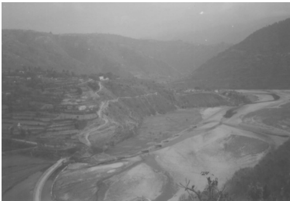
Downstream end showing photograph of 12MW Jhimruk Hydropower Project
