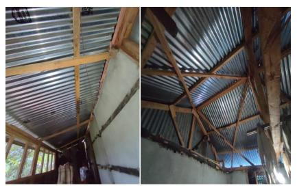
Figure 12: Inadequate rafter and Purlin in roof truss
