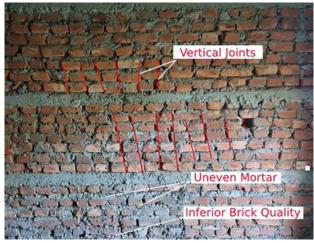
Figure 11: Vertical joint in brickwork
