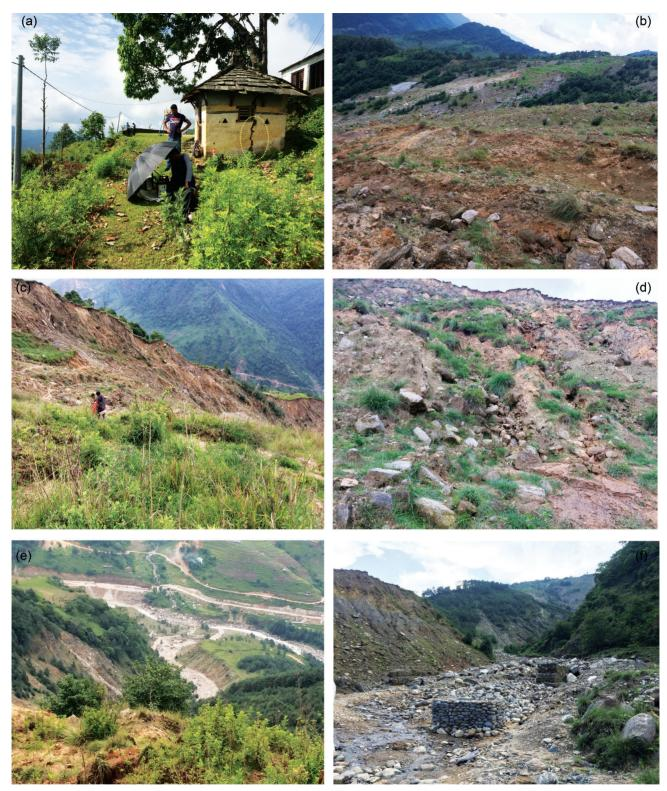
Fig. 4: (a) Cracks on the temple are present in the crown part (b) Large scrap present at the main body (c) Active part of the landslide at the left flank of the body (d) Several gullies and seepage are present at the main body (e) Downslope view of the toe and (f) Thick debris and overall landslide view from the toe area.
