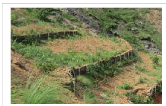
Fig. 6: Landslide mitigation measure at the source area.
