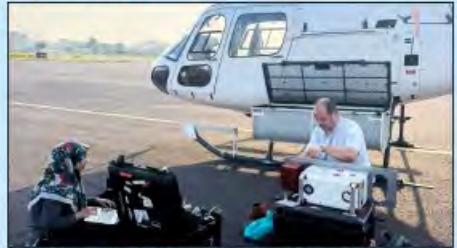
Expert team setting up the LiDAR sensor and receiver before conducting airborne LiDAR survey
