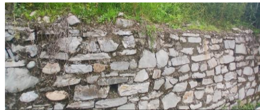
d) Dry masonry retaining wall
