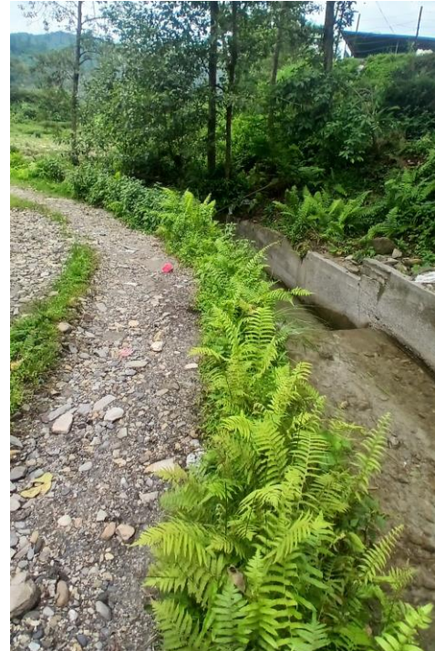
b) Concrete channel to convey Duhuni Khola
