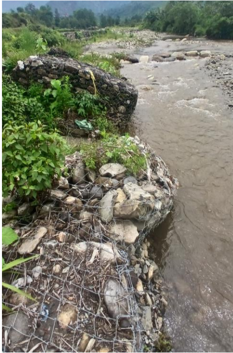
a) Gabion wall in the verge of failure at the right bank of Kali Khola
