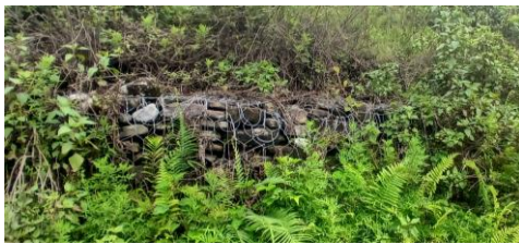
c) Bulging gabion wall
