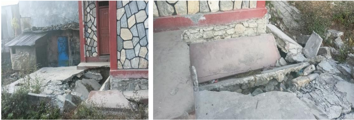
Figure 6: Picture of Sinkhole Affected Building
