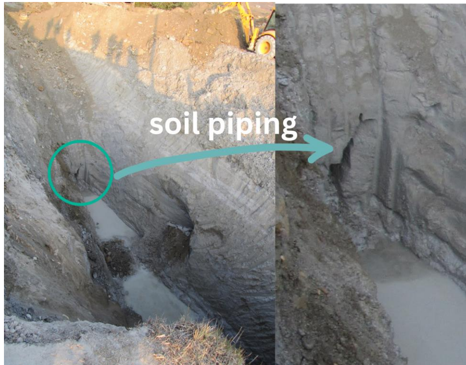
(c) One of the sinkholes revealed the presence of a soil piping
