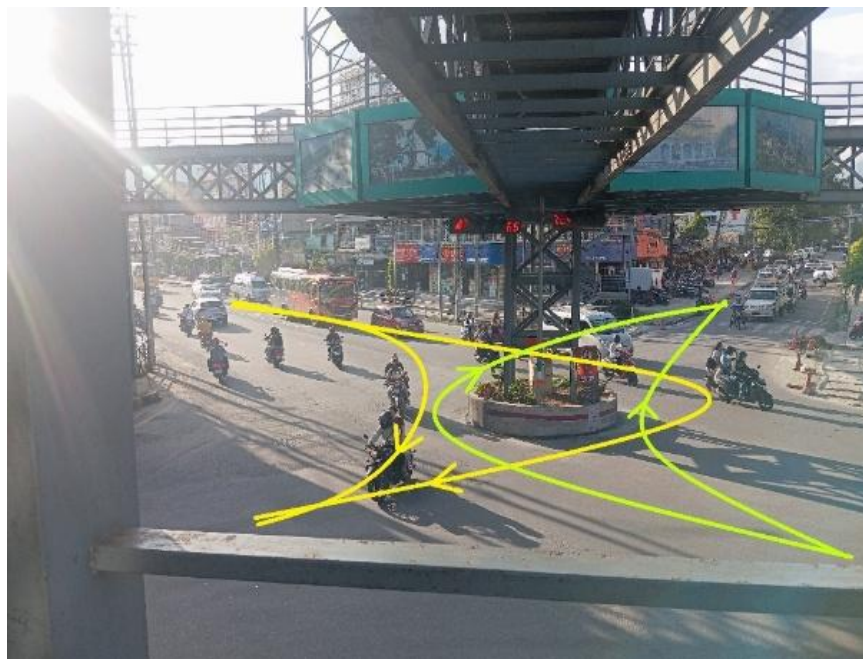
Figure 14. Confusion on Turning due to Pillar and markings
