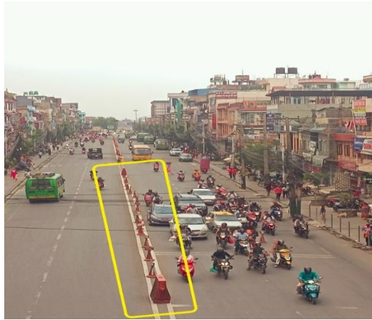
Figure 17. Plastic Cones Median Regulating Traffic in Eastern Leg
