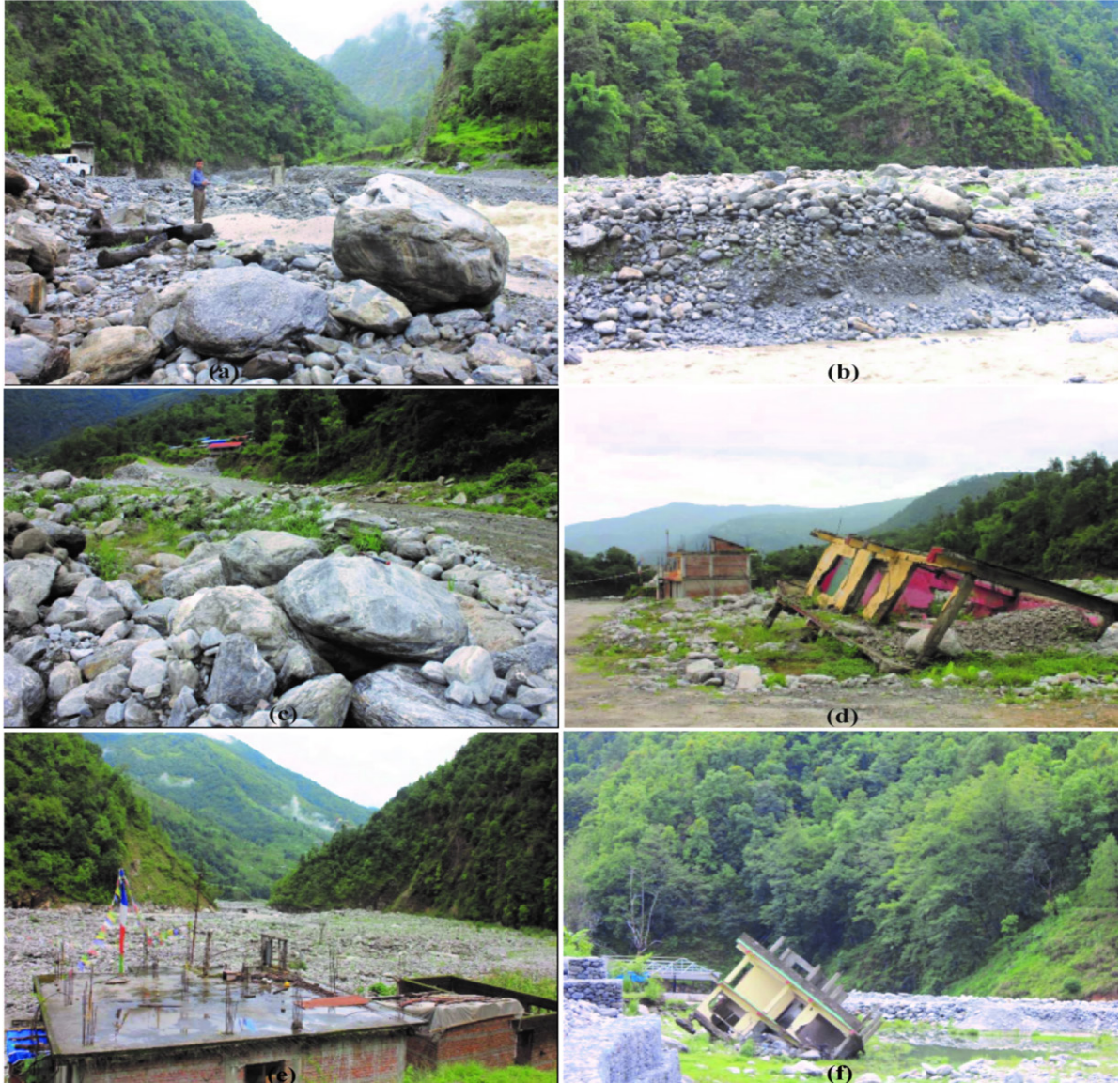
Fig. 8: Debris flow, houses damaged and buried between Ambathan and Ganeshi (a) Boulder of the flood erosion at Ambathan, (b) Inverse grading of the debris flow deposits south of Halde, (c) Road on the boulder bar at Kiul, (d) Destroyed houses at Ganeshi, (e) Houses partially buried by debris flow at Halde, (f) Damaged house at Kiul.
