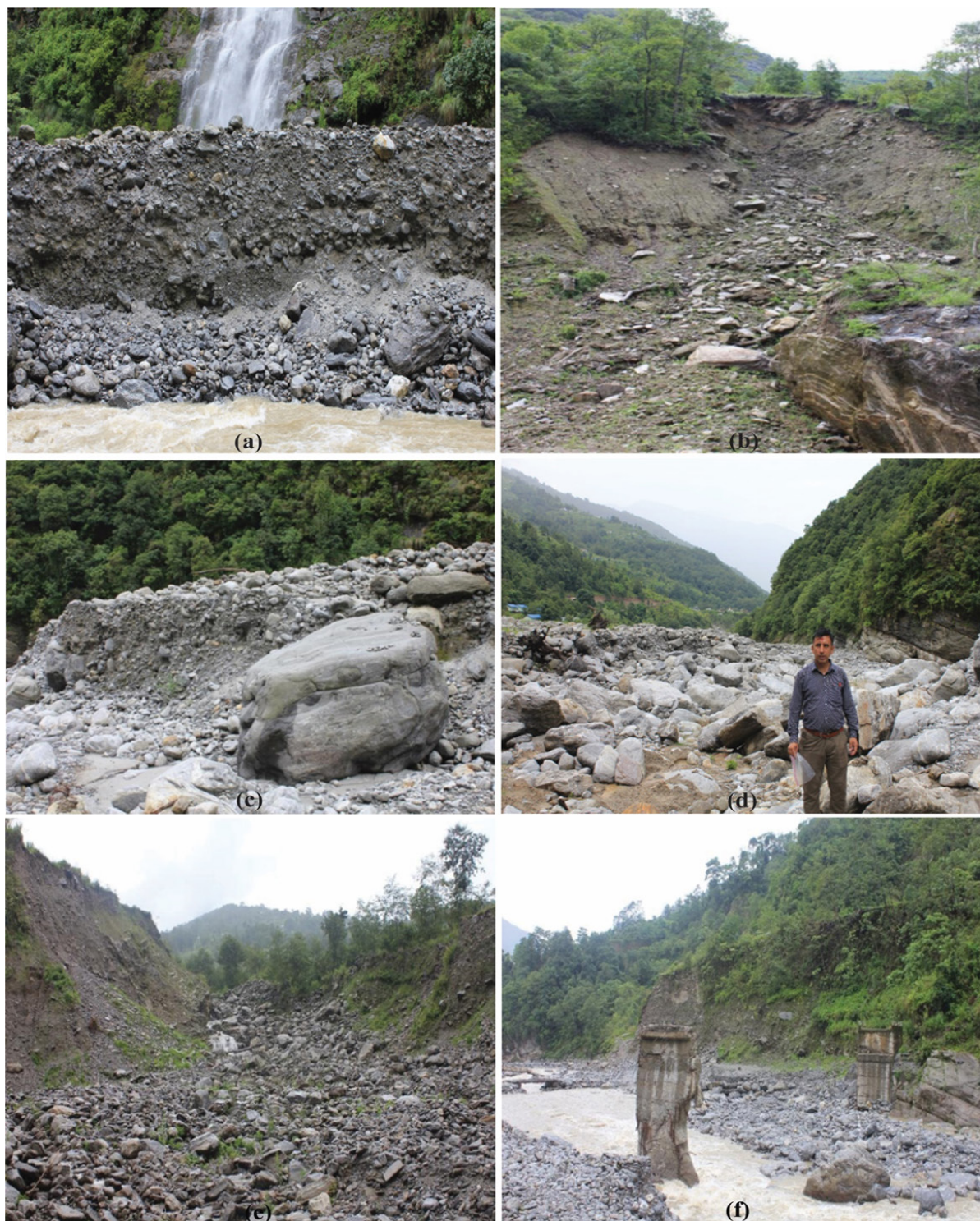
Fig. 7: Debris flow, landslide and flood related observations between the headworks and Ambanthan, (a) Deposits seen at the road section, (b) Landslide of colluvial soil on weathered gneiss, (c) Debris flow cliff (4m), (d) Debris flow remanent at Timbu, (e) Cut height of debris at the bank of tributary, (f) Ambathan road washed out bridge.
