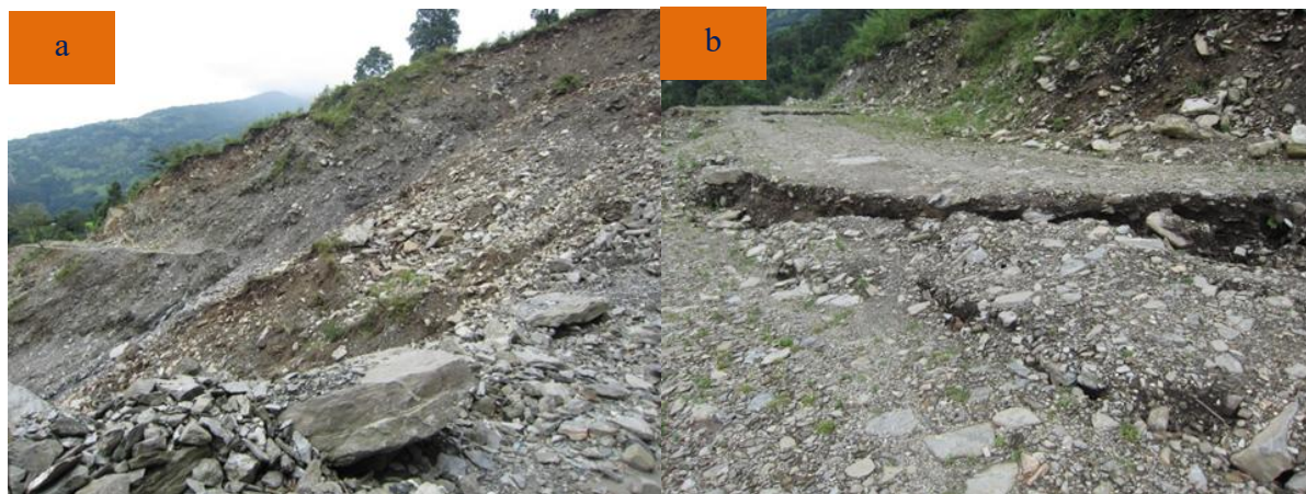
Fig. 7: (a) Slope failures blocking the foot-trail and (b) land subsidence (approximately 20 cm) near the landslide area
