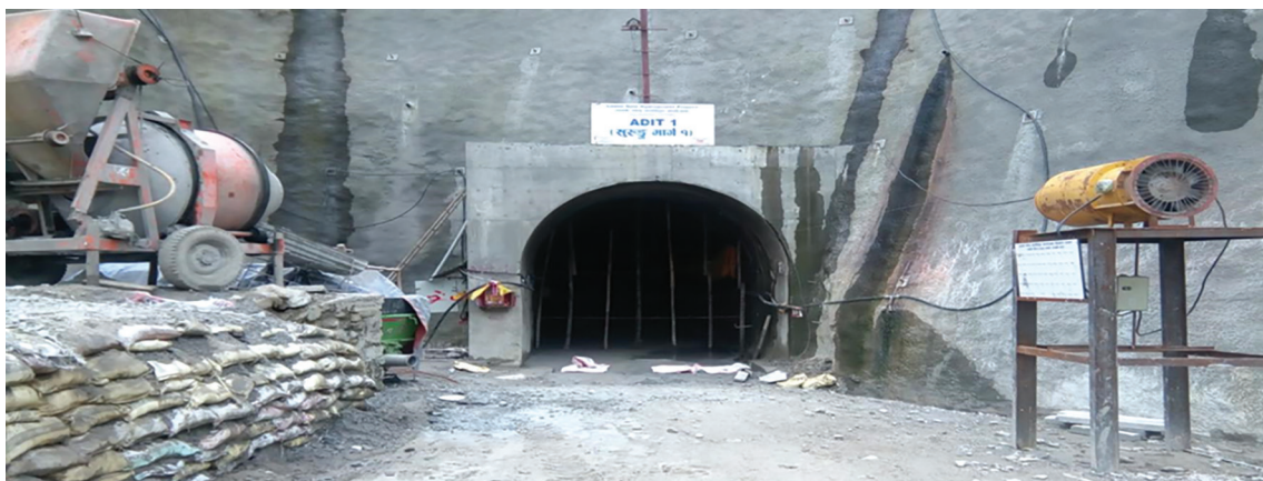
Figure 7: Inverted D shaped tunnel of Lower Solu hydro-project
