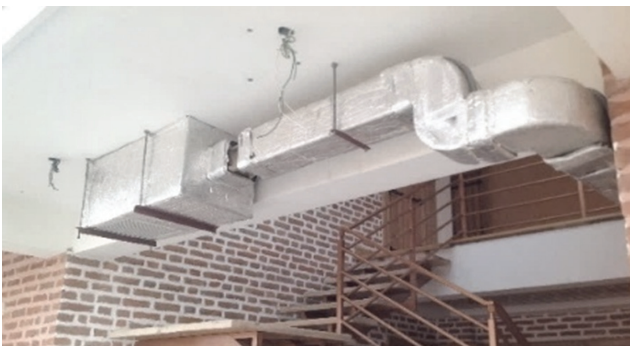
Figure 8: Duct to supply hot and cold air
