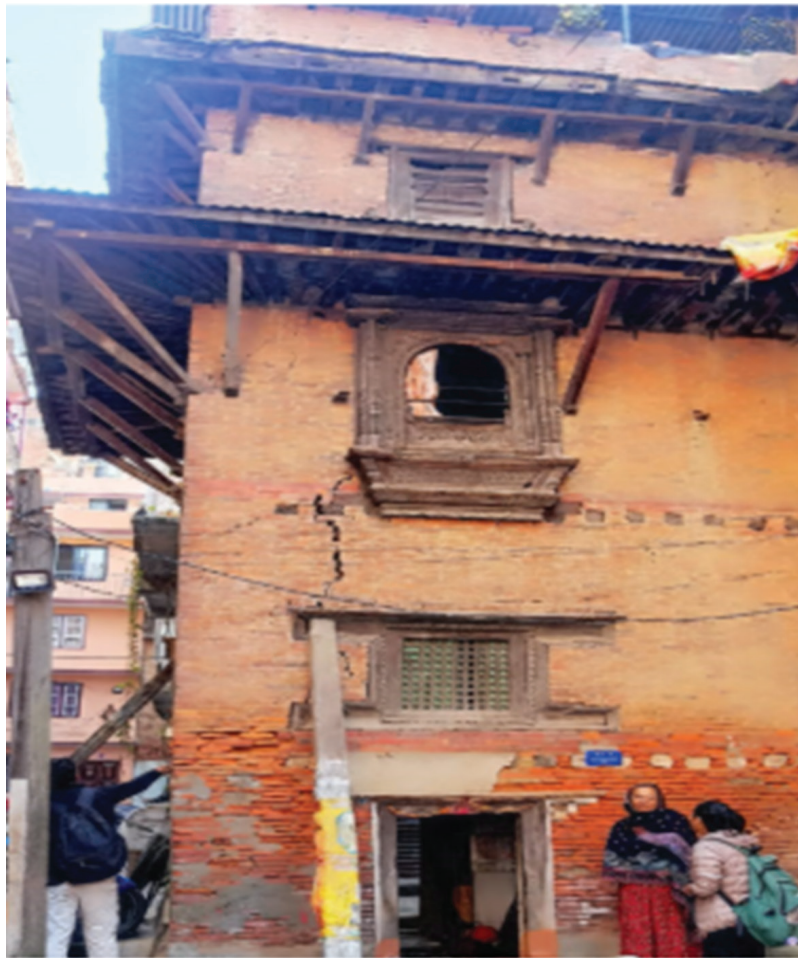
Figure 4: External view of the selected pre-1934 traditional masonry building in Patan.
