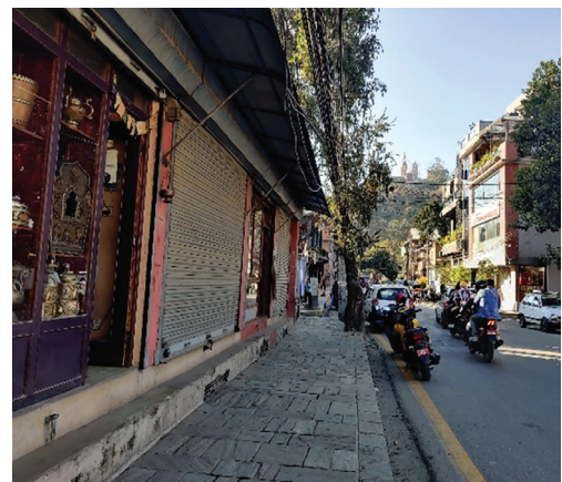
Figure 21: Lacks Proper Separation
