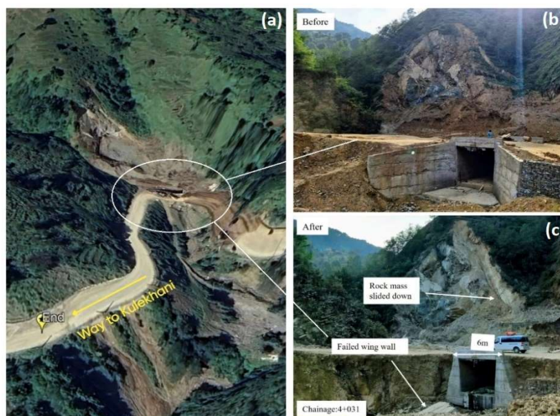
Figure 9: Pictorial comparison of before and after the monsoon at different chainage; (a) Satellite Map of the alignment part, (b) Before monsoon picture of chainage 4+031, and (c) After monsoon picture of chainage 4+031
