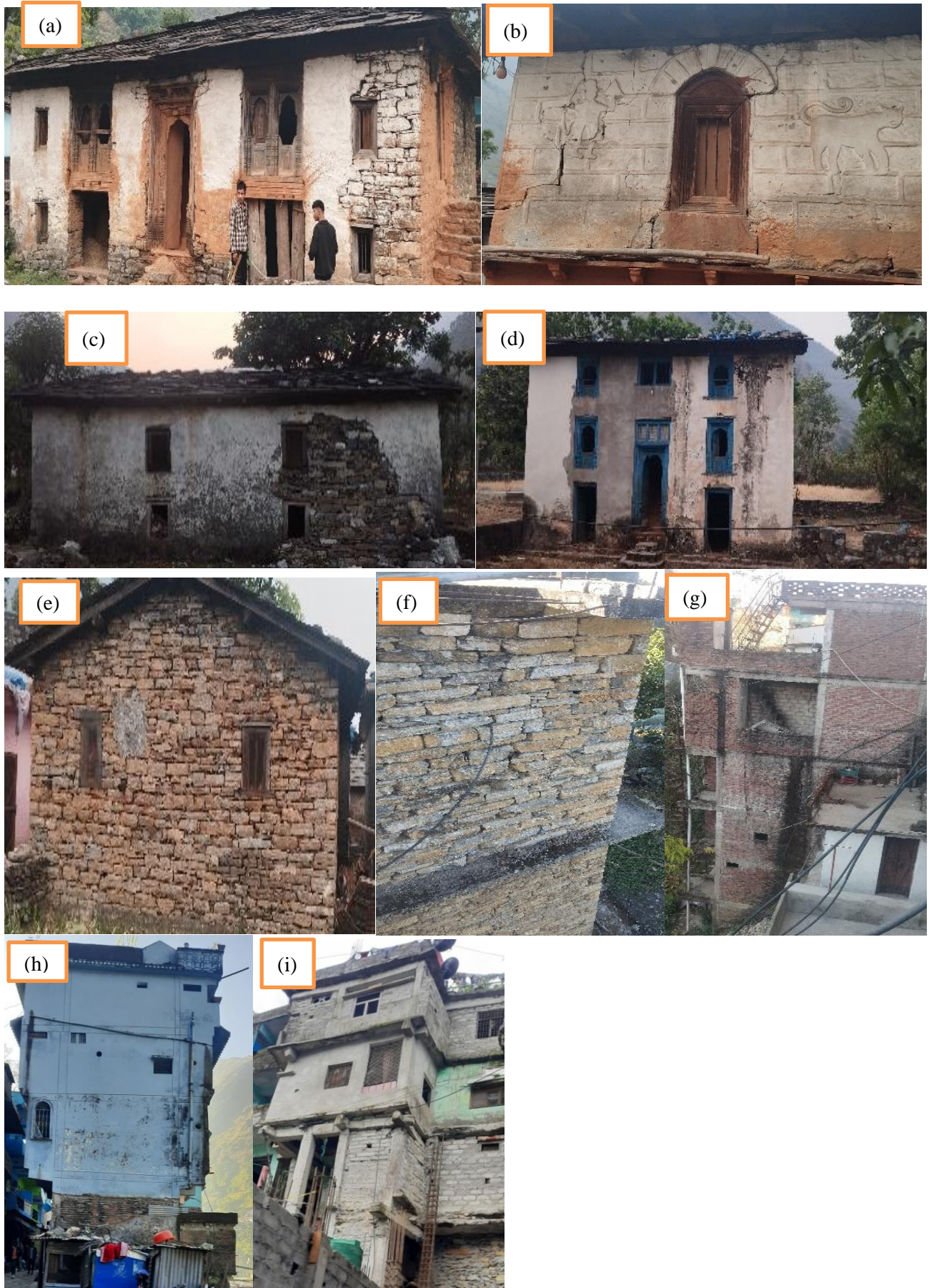
Figure 2: Common construction practice in structures in Darchula
