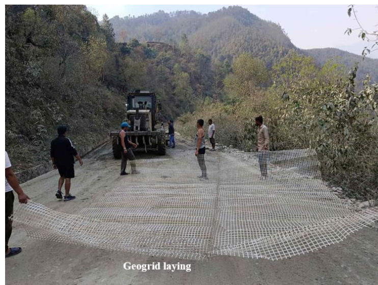
Figure 2. Placement of Geogrid (40/40Q Polypropylene, bi-axial 16kN/m, Tensar Product)
