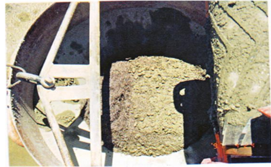
Photo 3 Condition of the macro-mix of pre-mixed
