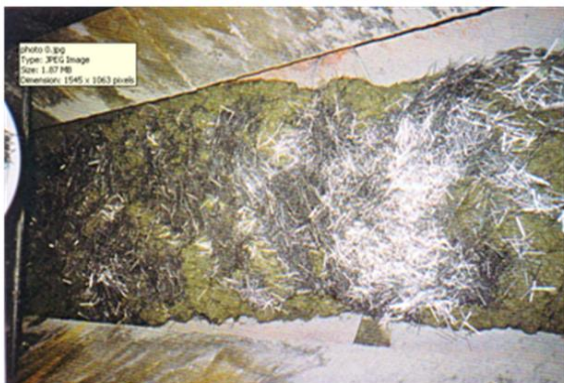
Photo 1 Condition of layered pre-mixed concrete and SF on conveyor-belt before charging
