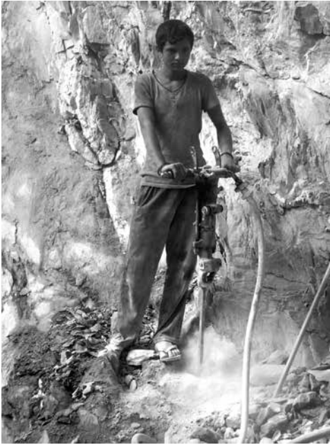
Picture 2: Hydraulic power tools using pressurized air-hoses are used to break up and destabilise the rock structure so that the man-power can remove rubble by hand. These machines require diesel fueled compressors, there is always a lot of spillage and ground contamination which often leaks into water courses or the water courses are ultimately destroyed. The young works are not provided with the appropriate protective clothing and many are seriously injured during the work - Dolpa © Ian Wall
