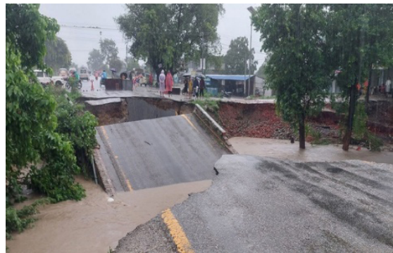
Figure 16 Culvert collapsed at Bedkot, Kanchanpur district along East-west Highway
