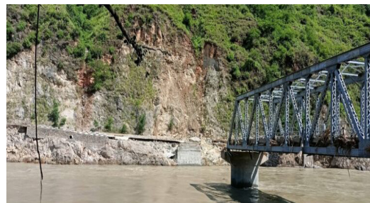
Figure 7 Bridge connecting Sindhuli and Ramechhap to Okhaldhunga damaged by the flooded Sunkoshi River, ( https://english.khabarhub.com/2024 )
