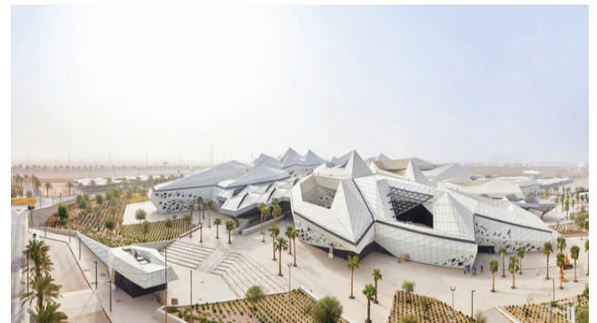
Fig. 1 KAPSARC (King Abdullah Petroleum Studies and Research
