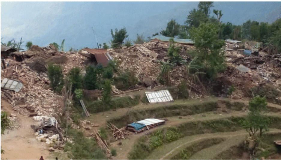
Figure 3: Completely Collapsed dry Stone Masonry Houses
