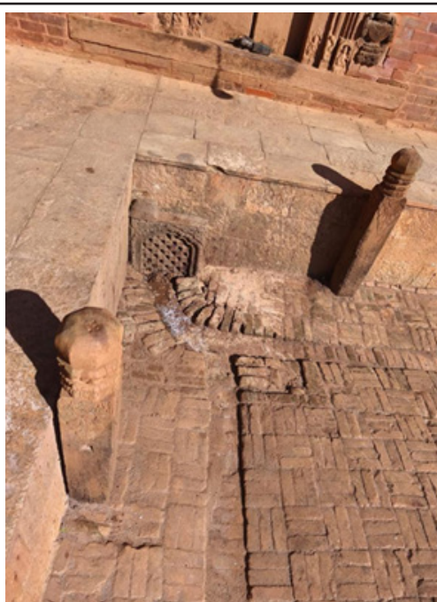
Fig. 12: Aankhijhyal gutter cover and gutter located in north-eastern corner of Mul Chowk
