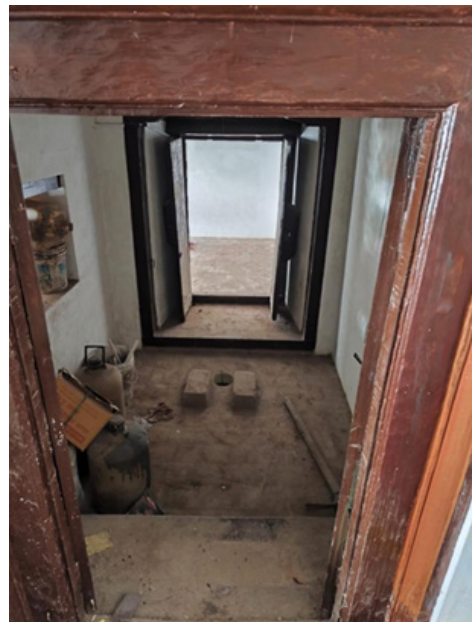
Fig. 16: Historical toilet basin no. 2 and bathroom or changing room in background
