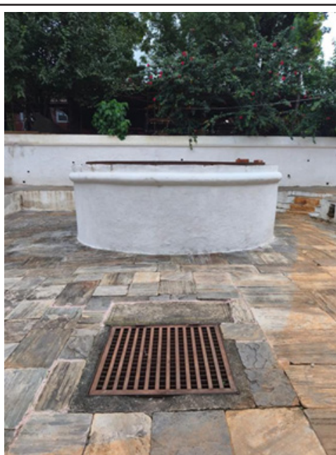
Fig. 8: Thulo Inar, and approach steps protected by an iron mesh cover
