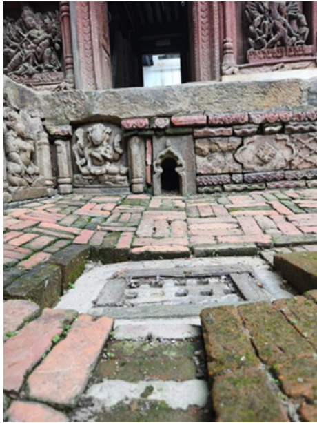
Fig. 13: Artistic niche below the plinth (back) and sewage inlet (front)
