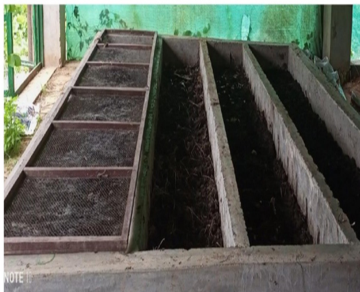
Figure 6. Vermicomposting tanks in car parking basement (Tripura University, 2019)
