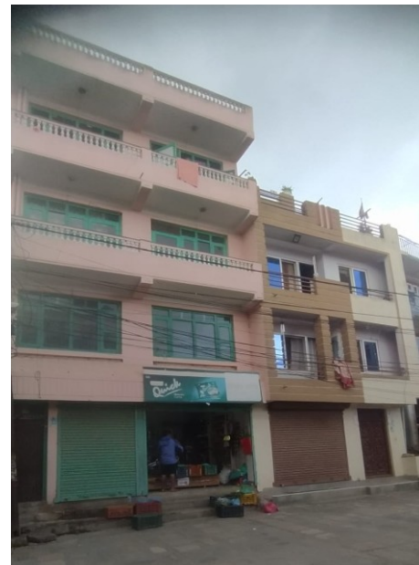
Figure 7 Completely New Construction
