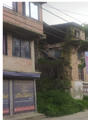
Figure 9 one section demolishes
