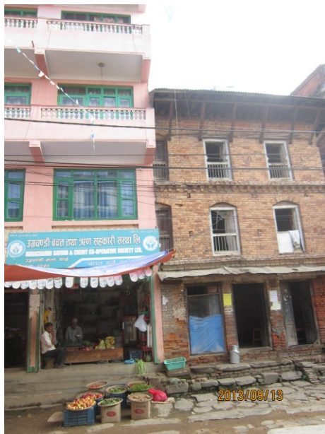
Figure 8 Partial New Construction
